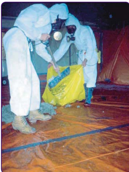
Type 3 removal half face respirators are no longer allowed for type 3 procedures
