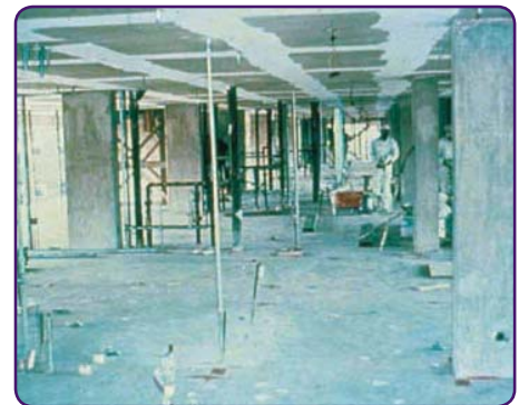
Removal of drywall joint compound now type 2 work.
